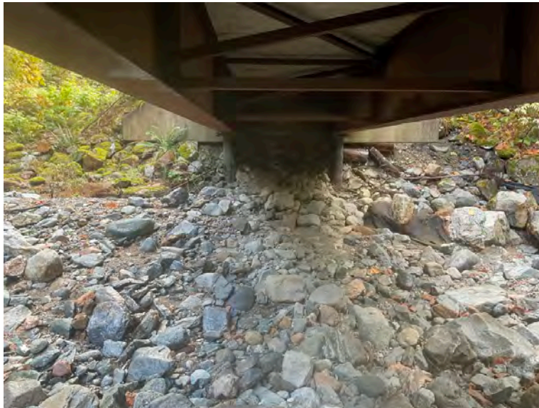
Left Bank Abutment when facing downstream
