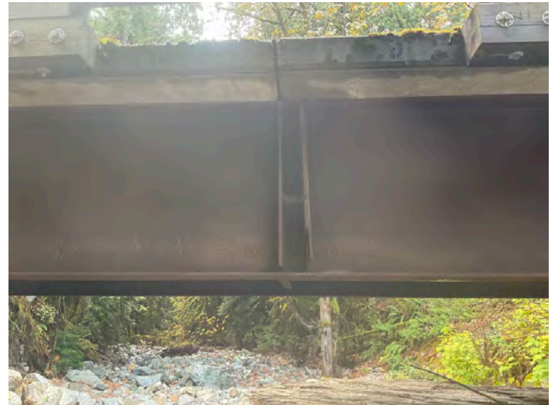
Upstream girder has stiffeners on upstream end
