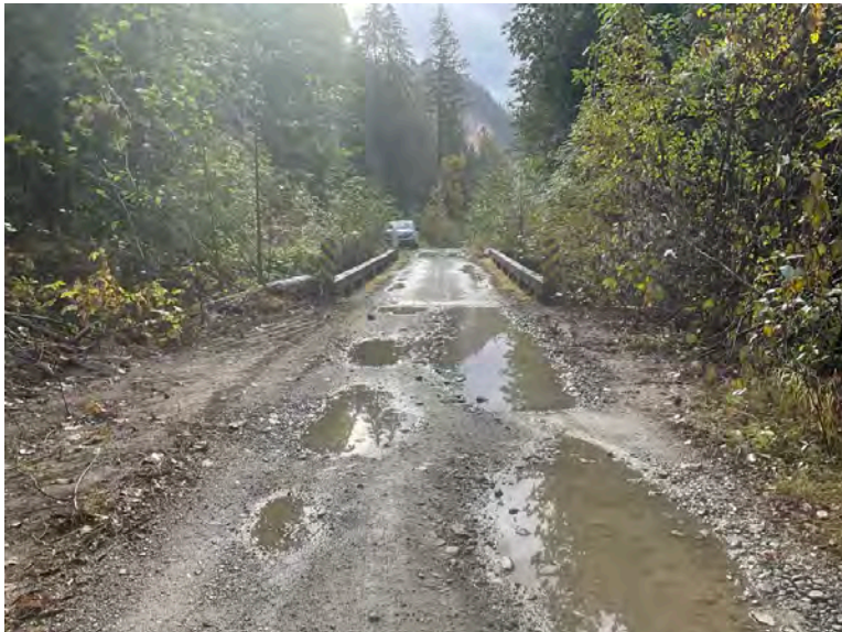
Approach from Right Bank when facing downstream
