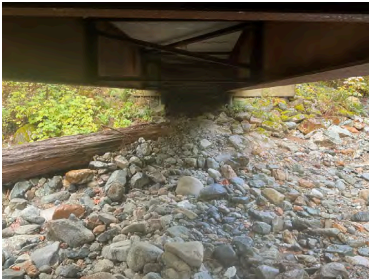
Right Bank Abutment when facing downstream
